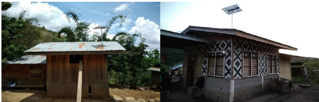
Diagram 7 : Roof-through Pole mounted installations on GI roofs
