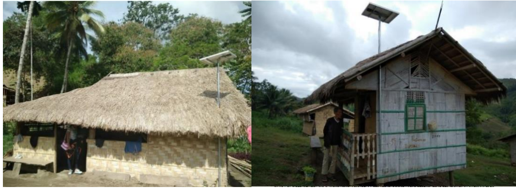
Diagram 8 : Roof-through Pole mounted installations on thatched roof
